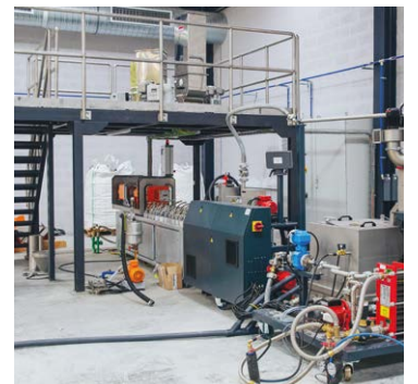
From top to bottom: the pilot laboratory building; Alexandre Gaspar, manager of the scale-up and new business sector at RAIZ; pre-mixed plastic and cellulose; biocomposites machine.
