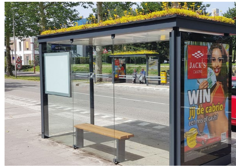
The Dutch city of Utrecht has put green roofs on 316 bus stops, most of them planted with succulents belonging to the Sedum genus, which are low-maintenance and flower nearly all year round.
