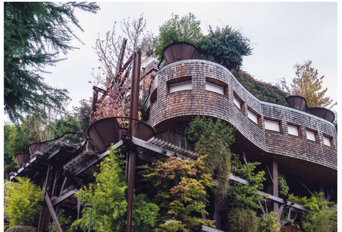
With the "25 Verde" complex in Turin, the architect Luciano Pia offers us an updated tree house.
